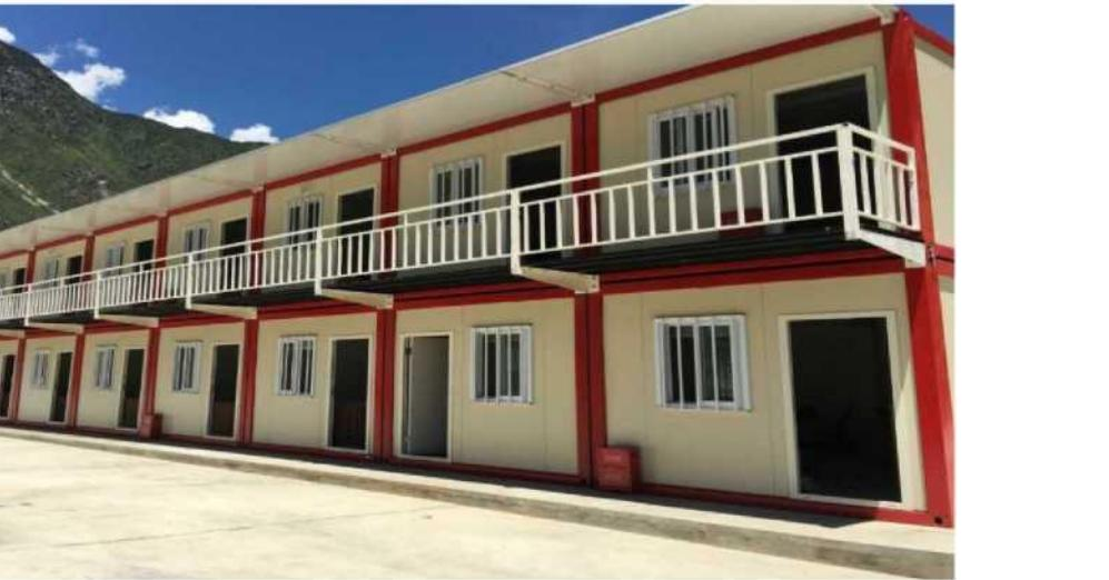
This product is customized and modularized with national standard steel. The amount of steel used is not less than that of the steel structure workshop. The color of the skeleton steel can be customized according to the user, such as Snow Mountain White, Zhongjian Blue, Construction Engineering Red, Engineering Gray, etc. Computer color matching, the frame is sprayed after pickling and phosphating, and the anti-rust and environmental protection grades meet the national standards.
